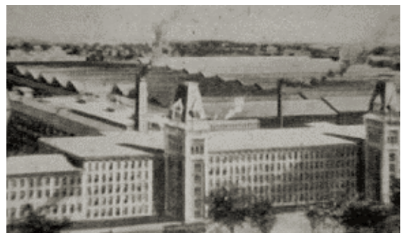
Social Mill complex after the fire
