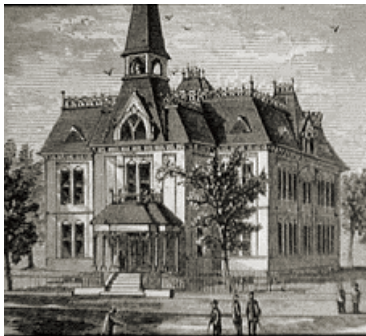
Woonsocket High School after the fire
