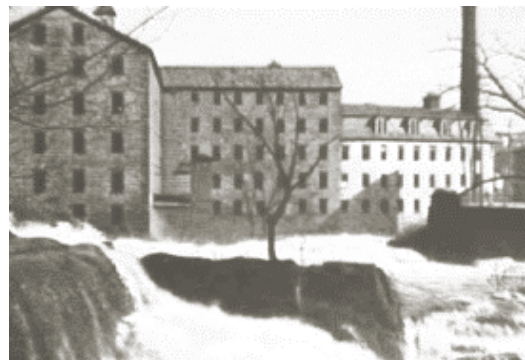
George C. Ballou Mill after the fire
