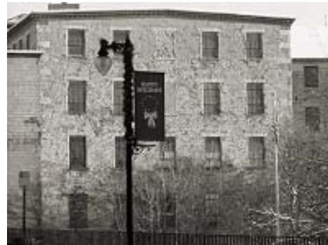
Harris Mill # 4 on Main Street as it appears today
